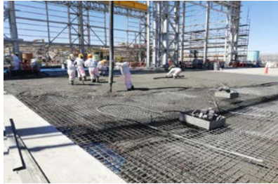
Heavy, labor-intensive traditional reinforcement
